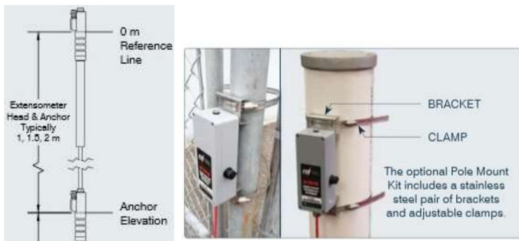
Figure 5.11. Installation of a Vibrating Wire Inline Extensometer and Single Channel Vibration Wire Data Logger
